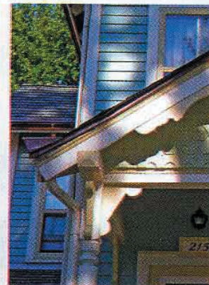
Repairs to Victorian details like gingerbread trim and shingle imbrication often measure a restoration's depth.
